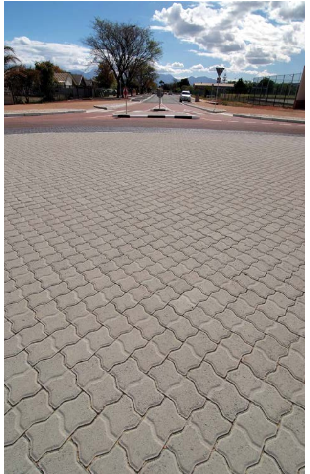
Worcester Traffic Circle- 203 x 102mm Grey Interlockers
