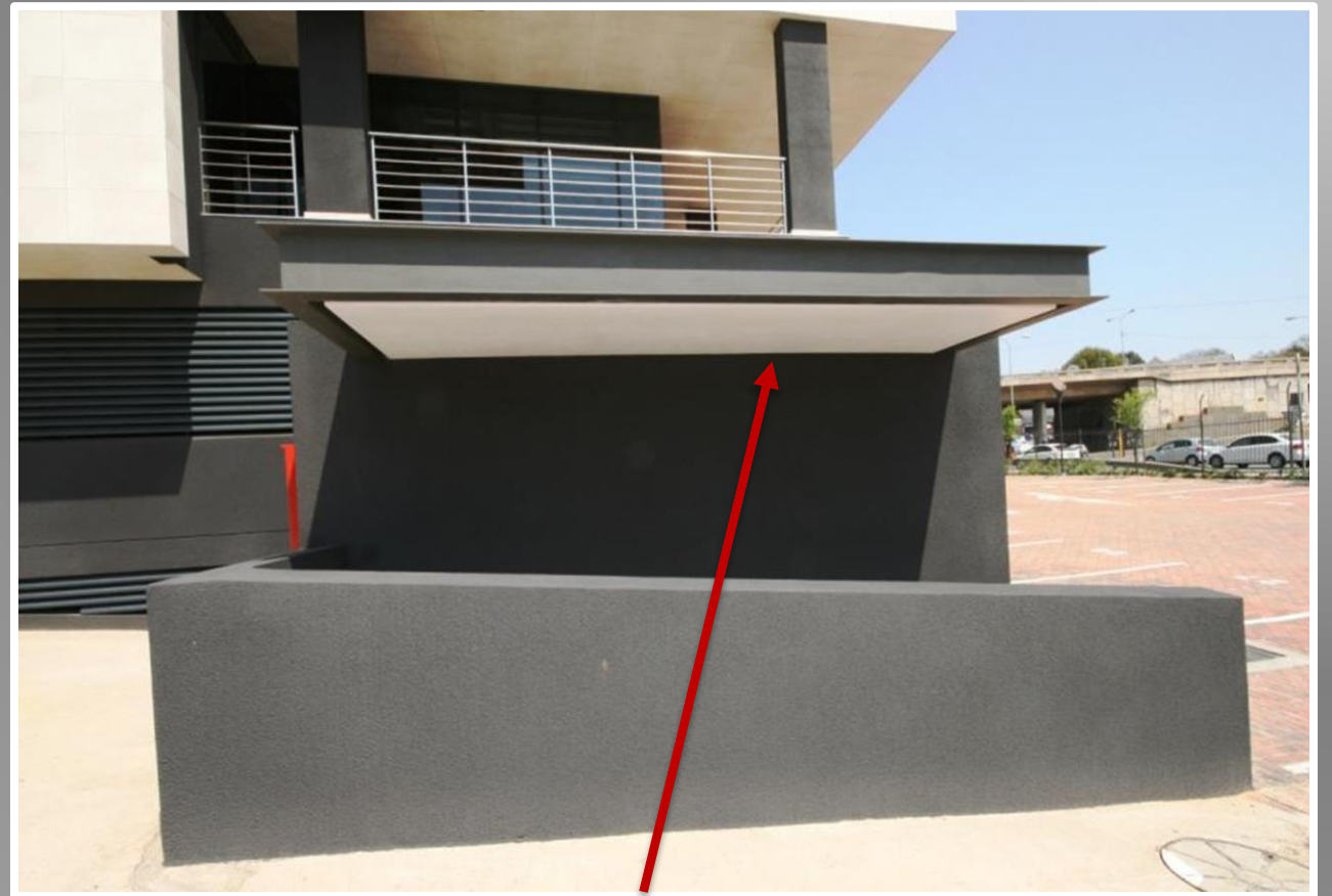
Decolite I beam and ceiling
