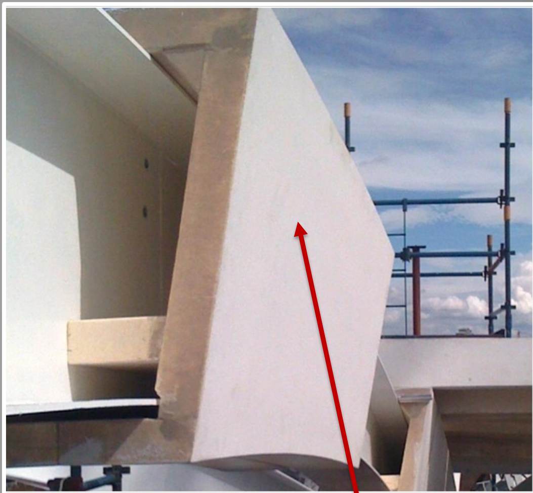
Decolite Cladding to I beam
