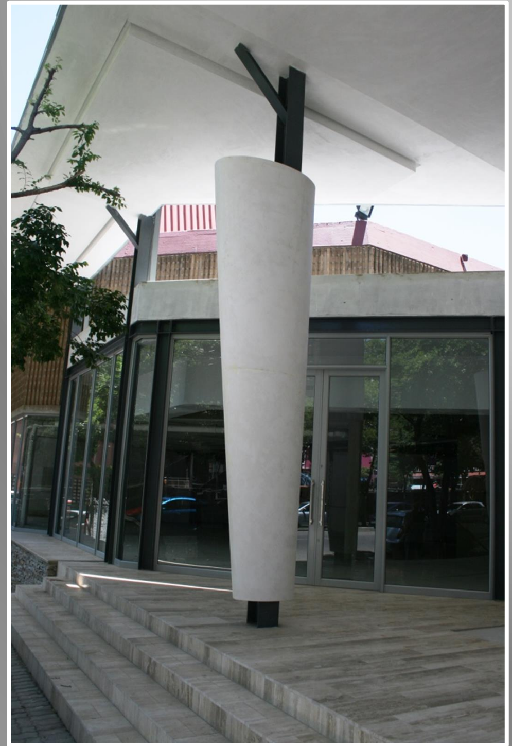
Decolite Cladding to I beam
